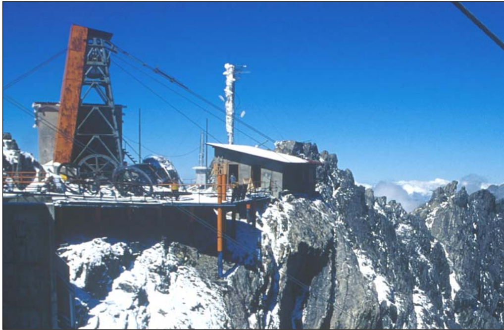
East side of the MARS building with the entrance door on the right. The microwave instruments use the completely unobscured view toward north through the right wall (in shadow).
